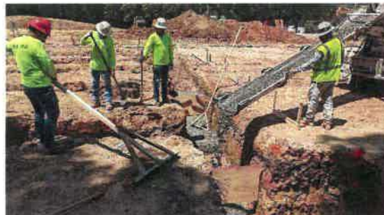
Picture 2: Indicates lean concrete backfill after undercutting of unsuitable bearing material.
