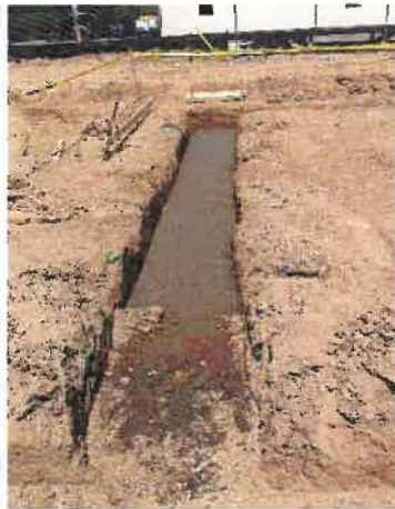
Picture 1: Indicates lean concrete backfill after undercutting of unsuitable bearing material.
