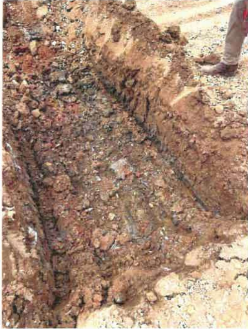
Figure 4: Test Pit Revealing Soft Soil Conditions
