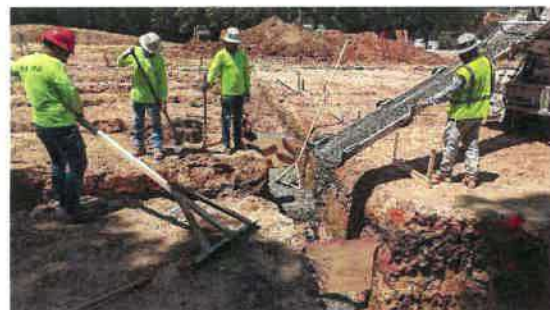
Picture 2: Indicates lean concrete backfill after undercutting of unsuitable bearing material.
