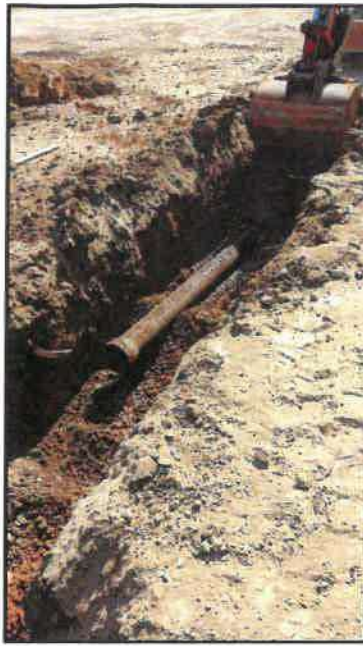
Picture 1: Indicates abandoned utility within footing requiring undercut to suitable soil (column B.5 0.6/0.8)
