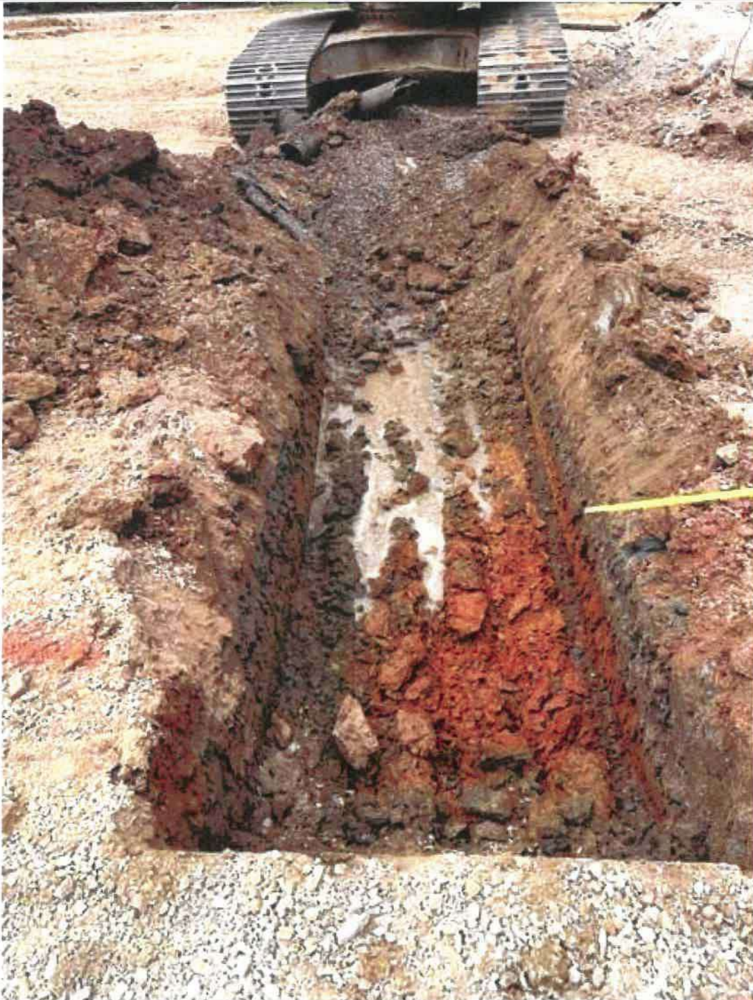
Figure 2: Test Pit Exhibiting Perched Water Condition
