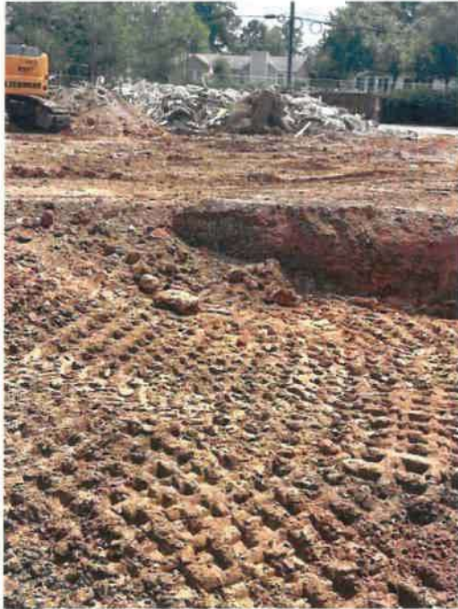
Figure 1: General Undercut Area of Observation Looking East
